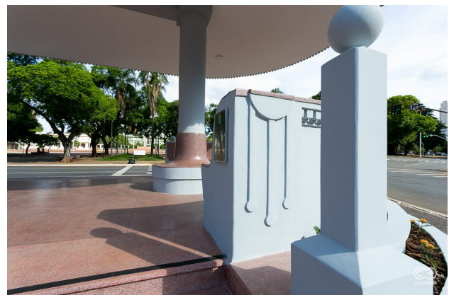
Fig. 43 Coreto after renovation - 2020
