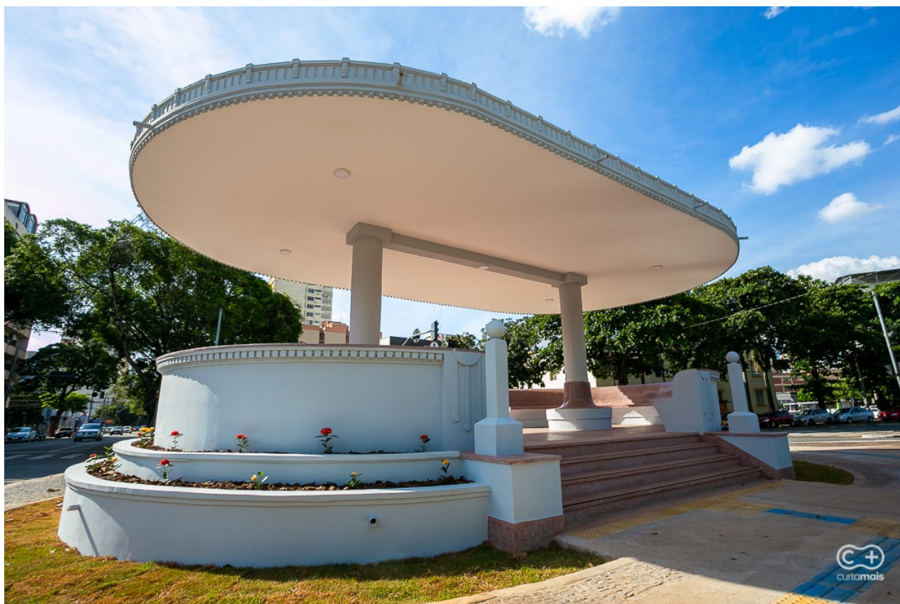
Fig. 41 Coreto after renovation - 2020
