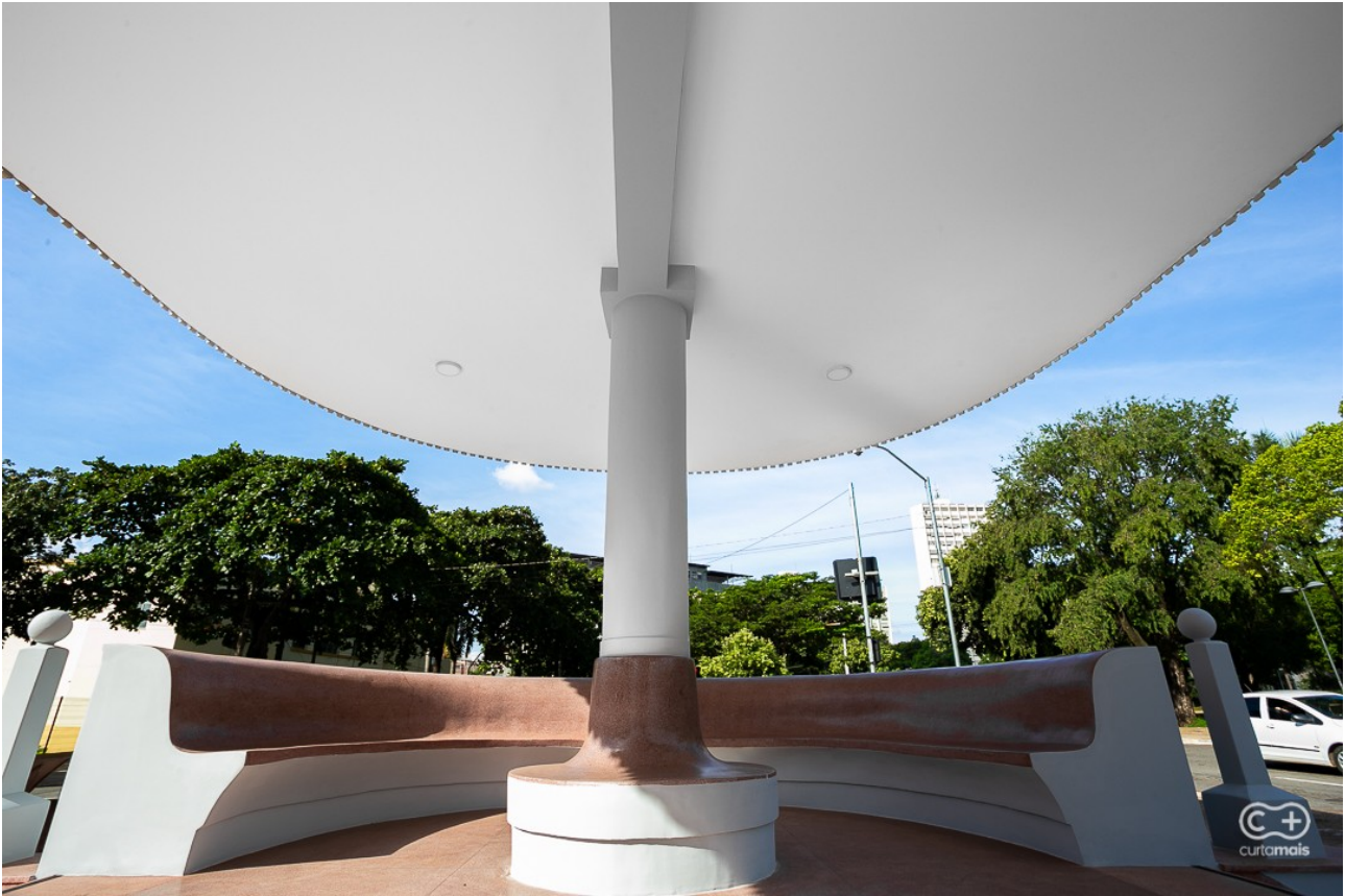
Fig. 44 Coreto after renovation - 2020
