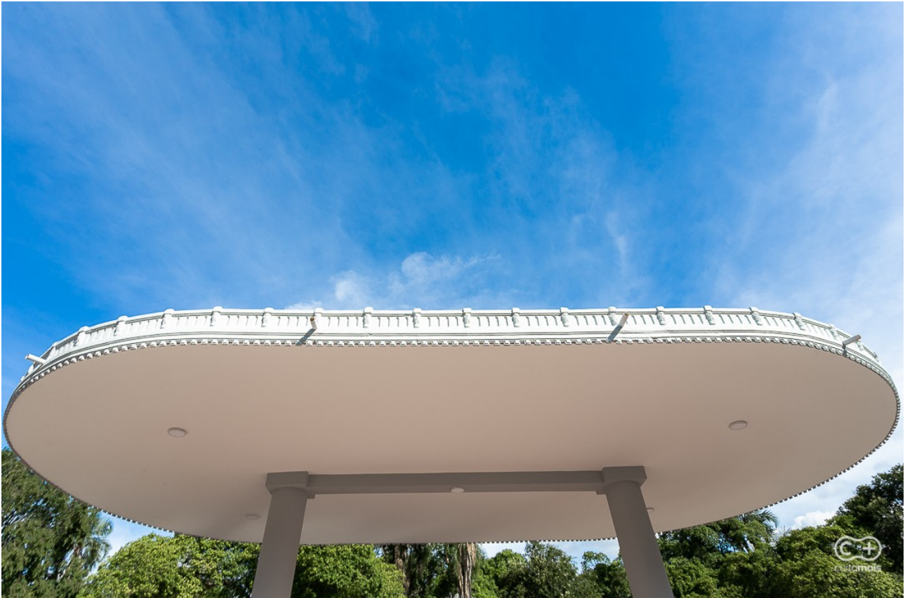
Fig. 42 Coreto after renovation - 2020
