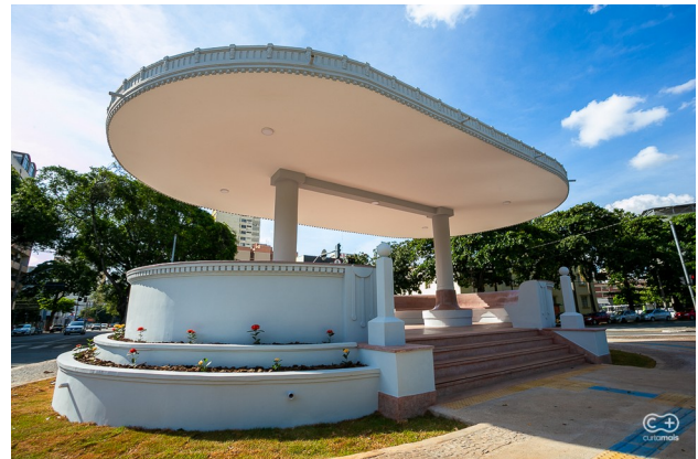
Fig. 41 Coreto after renovation - 2020
