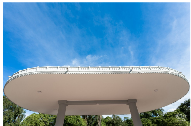
Fig. 42 Coreto after renovation - 2020
