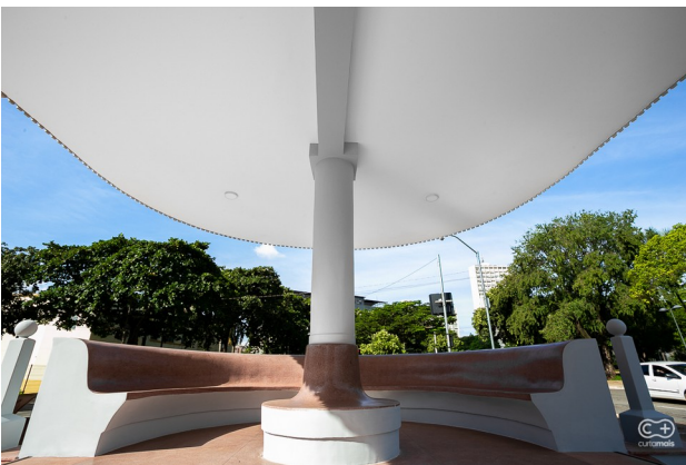
Fig. 44 Coreto after renovation - 2020
