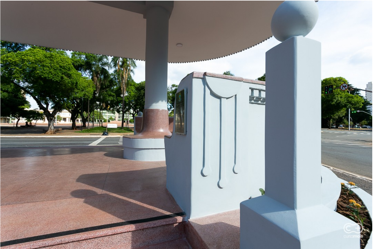
Fig. 43 Coreto after renovation - 2020
