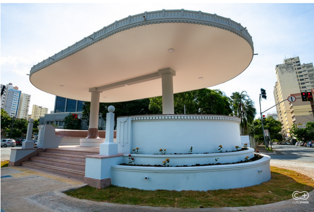
Fig. 45 Coreto after renovation - 2020
