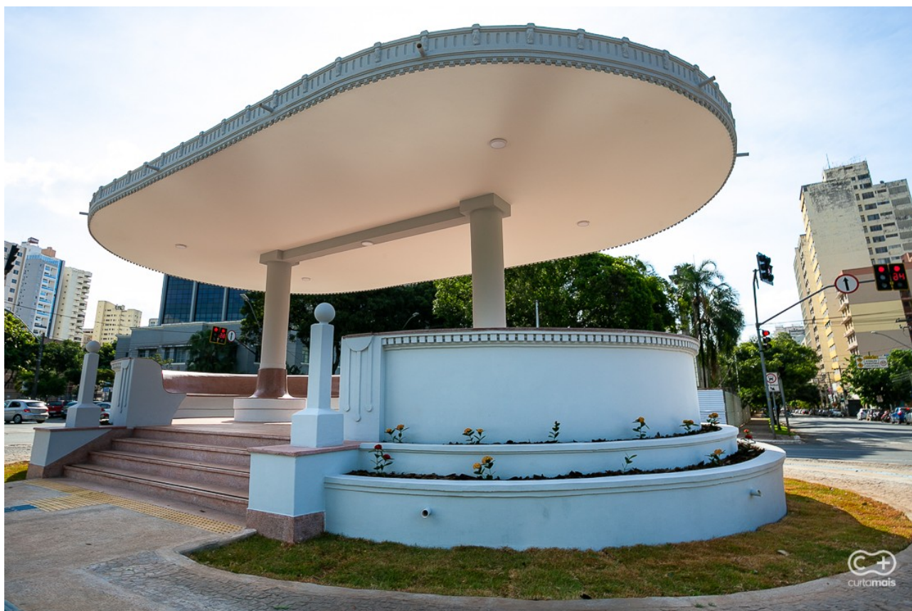
Fig. 45 Coreto after renovation - 2020
