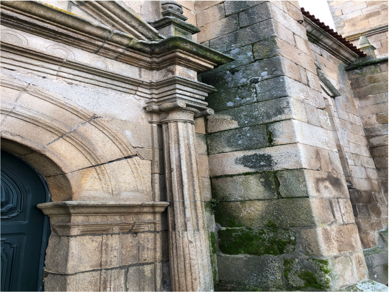
Fig. 23 North Portal - Column and Arch Detail
