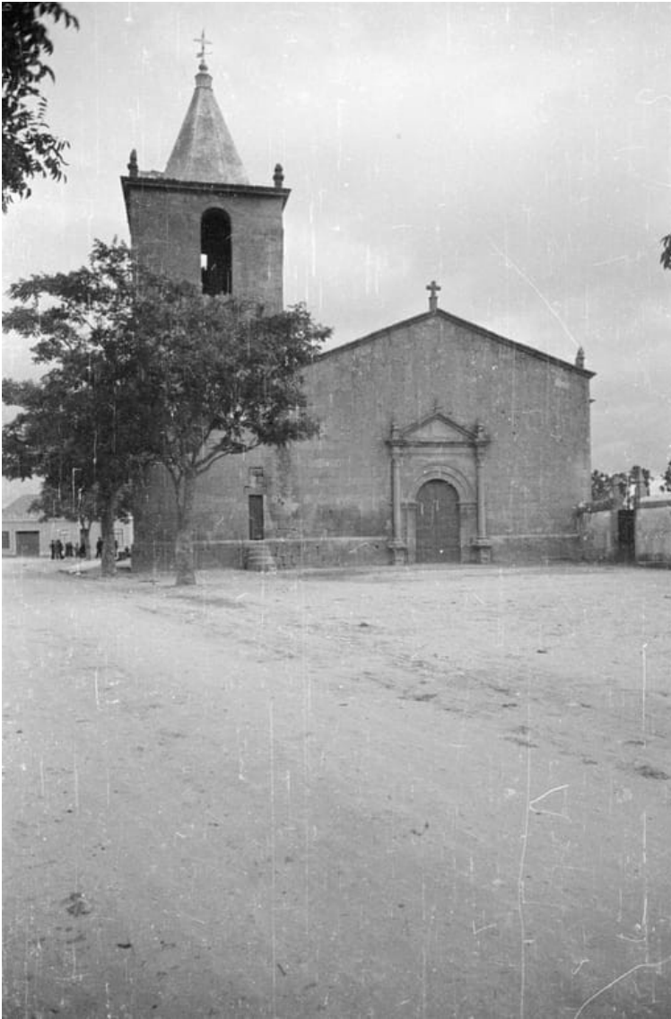
Fig. 7 Main Entrance of Escalhão Church
