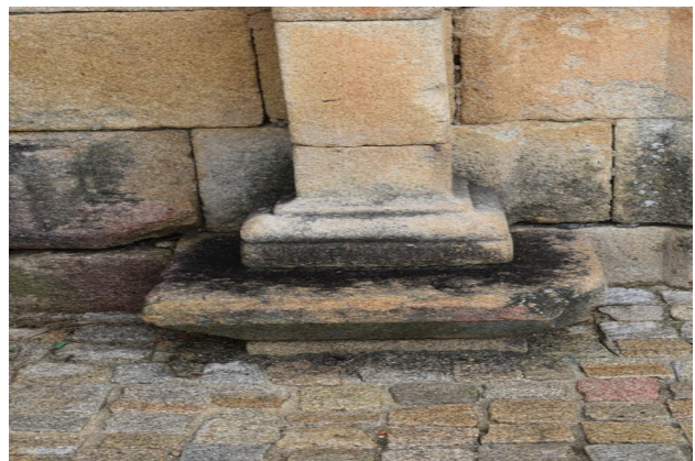
Fig. 39 2.03 South Portal's Column Base
