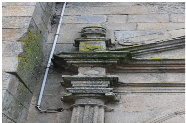
Fig. 28 North Portal, Entablature Detail
