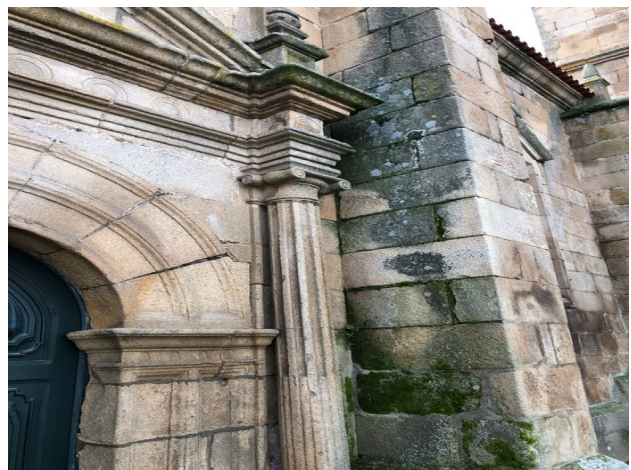
Fig. 23 North Portal - Column and Arch Detail
