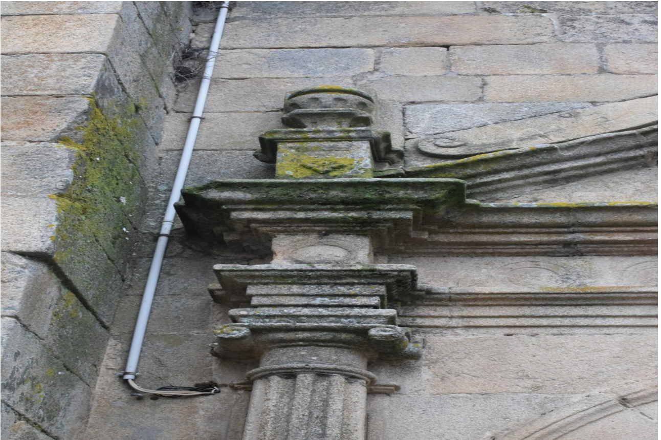
Fig. 28 North Portal, Entablature Detail
