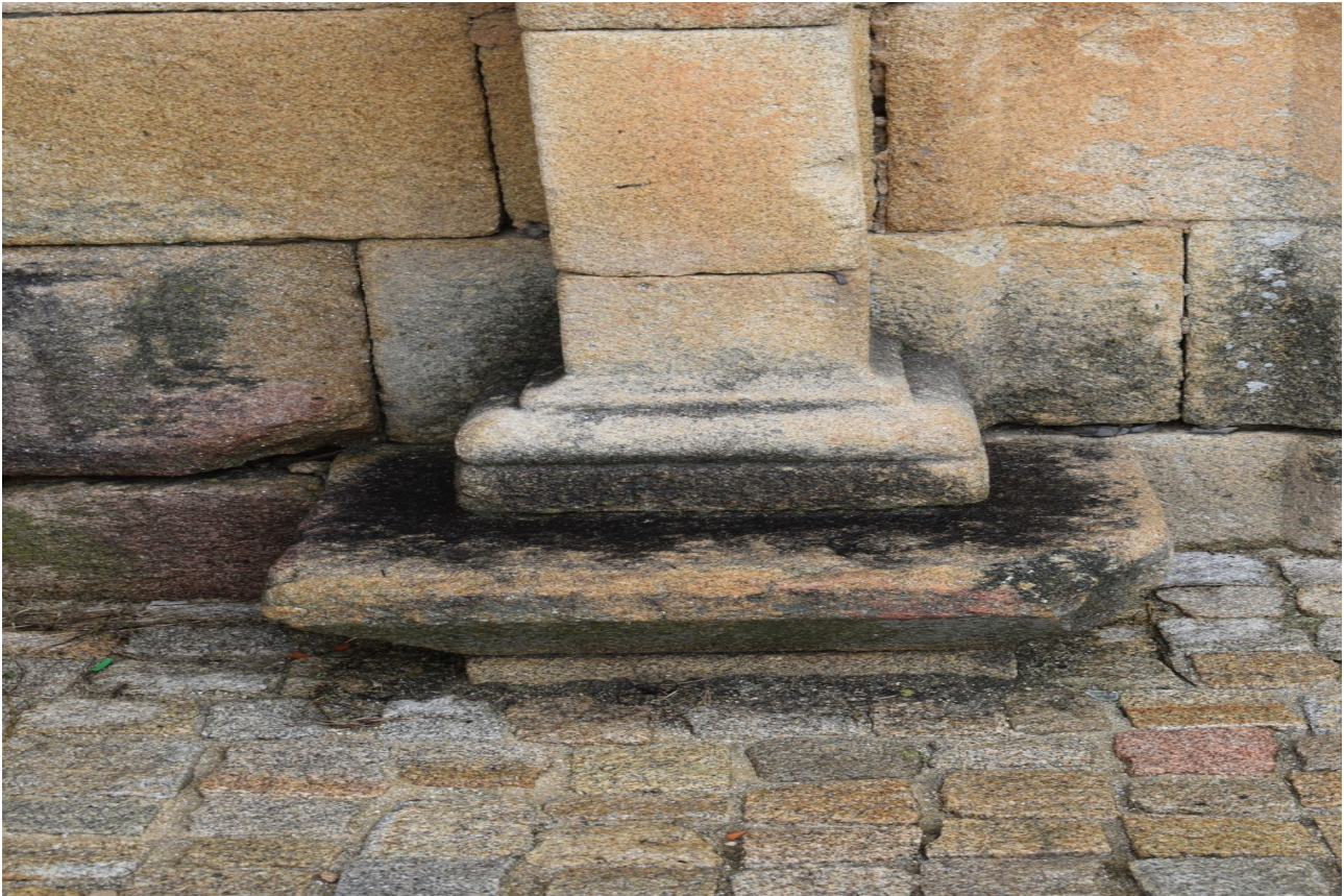
Fig. 39 2.03 South Portal's Column Base
