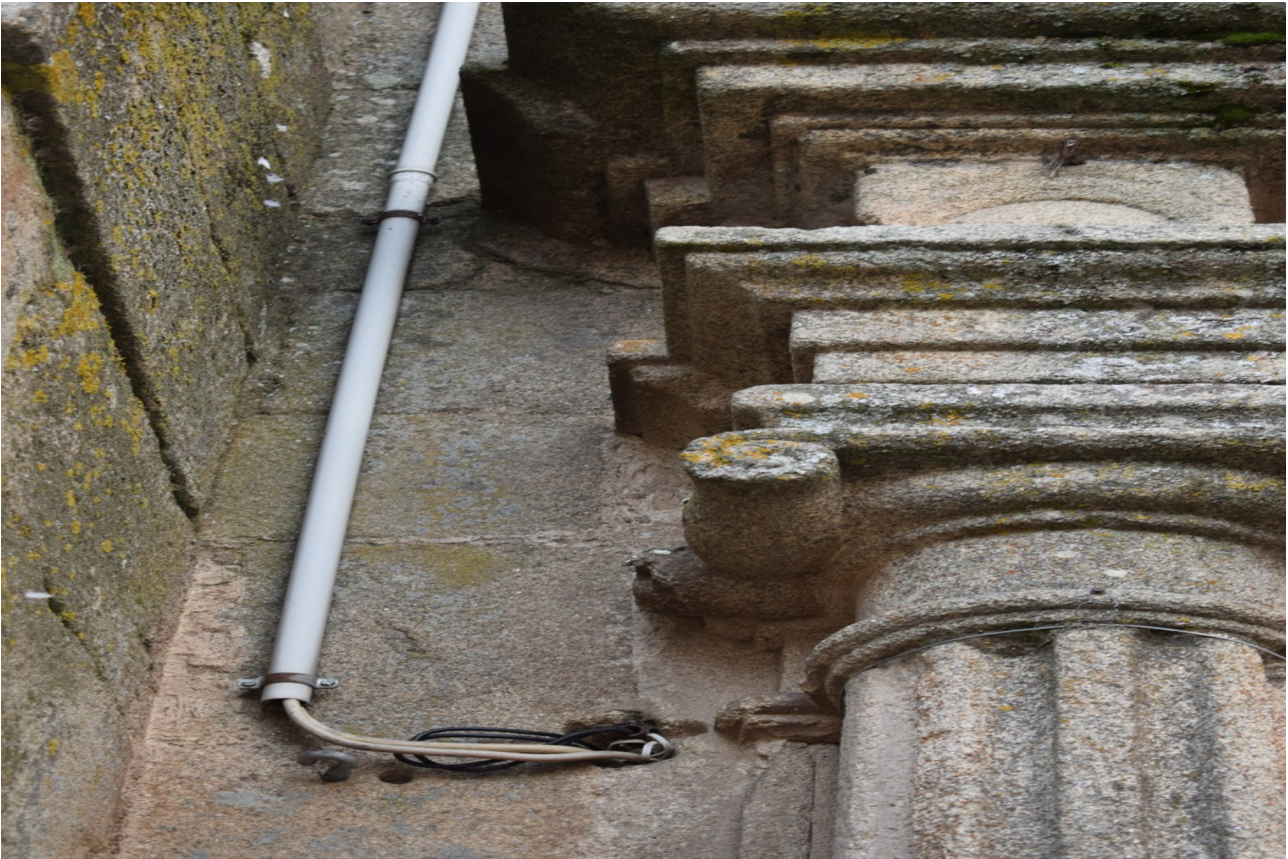
Fig. 29 North Portal, Column Detail
