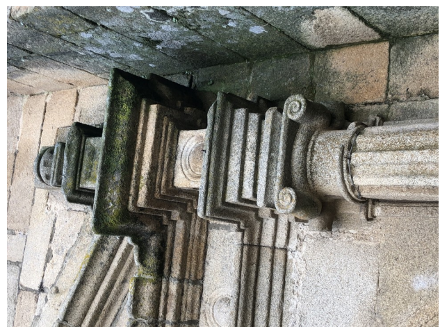
Fig. 24 North Portal - Entablature Detail
