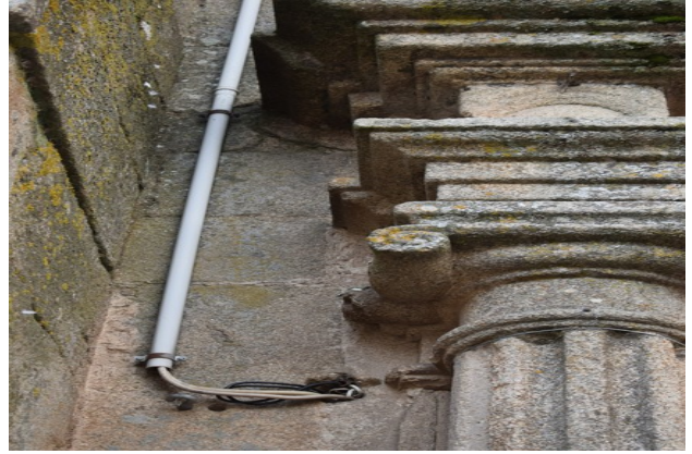
Fig. 29 North Portal, Column Detail
