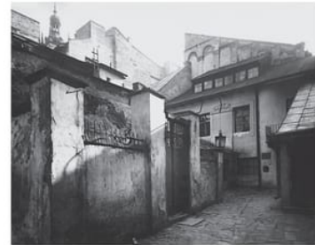
314. View from the west, state before 1939
