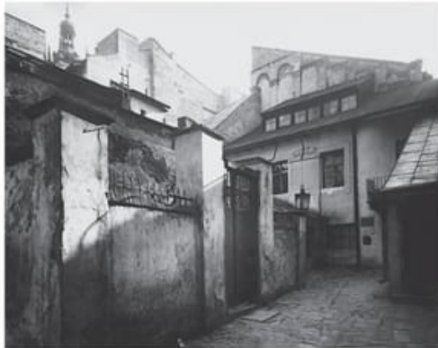
314. View from the west, state before 1939
